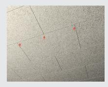
E: To open the access panel, press the Troldtekt acoustic panel lightly under the push release locks.
